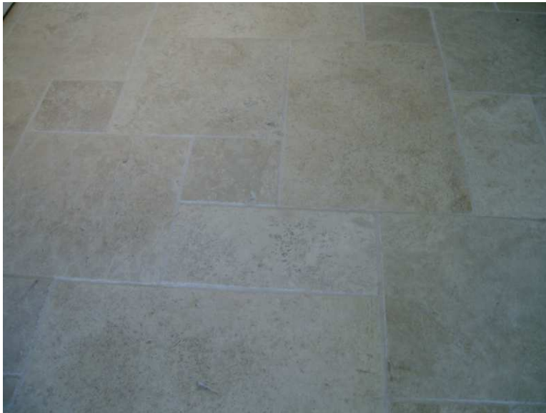
Ground level tiled Flooring
